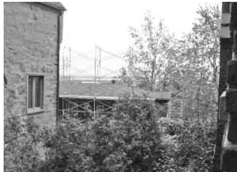
From Sunnyside looking south: new roof would reach close to top of scaffolding.
