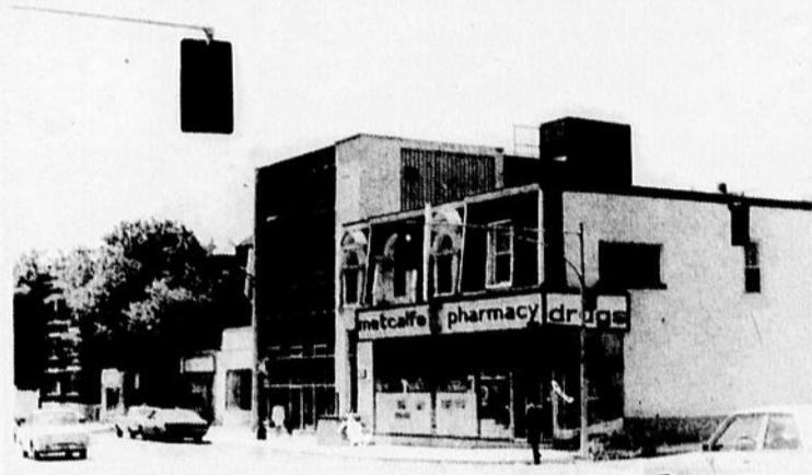
NEW LIGHTS INSTALLED: Frequenters of the area believe there have been fewer squealings of brakes and near collisions since the new overhead traffic lights, seen above this week, went into operation at the corner of Metcalfe avenue and St. Catherine street. The old lights, specially westbound, were difficult to see.
