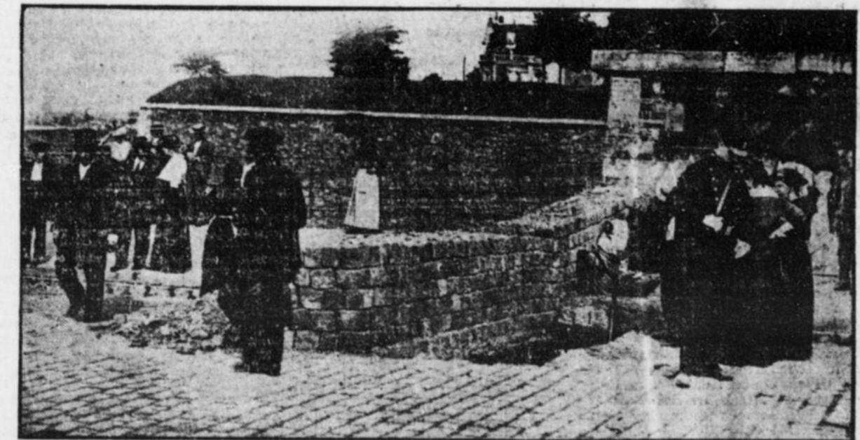
The photo shows a trench sunk in a street in the suburbs of Paris. The paving stones are piled in front of the hole, and strengthened by the earth excavated. Many of these trenches, and other types of barriers against the invader, have been made around Paris.
