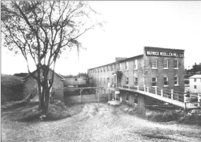
Mill number One, located at 274 Saint-Louis Street; in 1920, Cantin Industries became known as Warwick Woollen Mills Limited.
