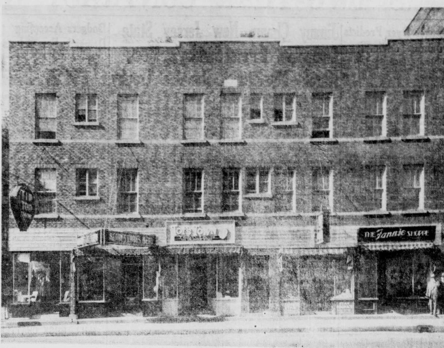
Seen above is the newly-renovated S. Echenberg building on Wellington street north. Containing stores and apartments, the building has had a complete exterior face-lifting, making it one of the most attractive establishments on Wellington street. The stores, left to right, are Tip Top Tailors, Henry's Ladies' Wear, Tot's Town, the Star Pharmacy, and The Fannie Shoppe. (Photo by Gerry Lemay).
