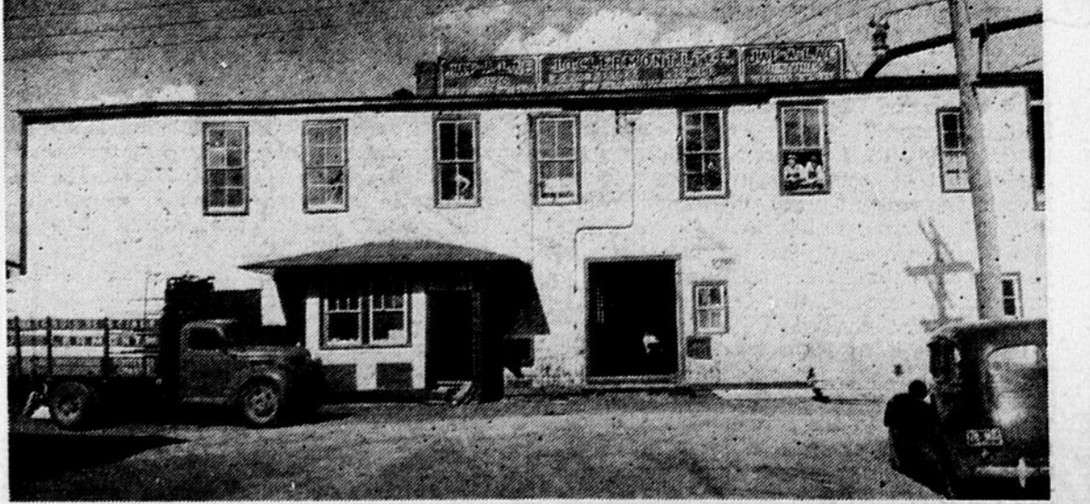
Above is the J. O. Clermont Factory in Valleyfield, which was lost in a fire which occurred early Sunday morning and resulted in a $50,000 loss and temporary unemployment for about 25 employees. The building was erected about 50 years ago. More than thirty firemen fought the blaze.
