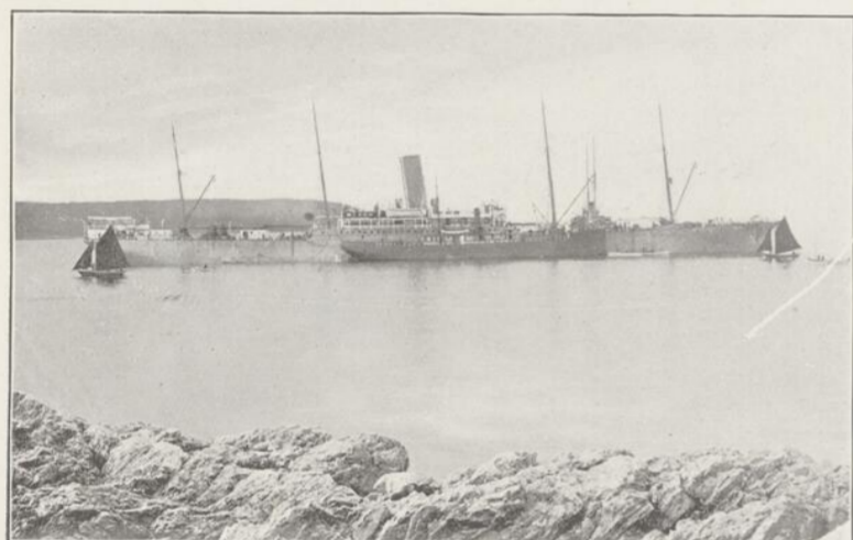
The cable steamer Colonia, taken at Canso, N.S., just before sailing to commence laying the new cable off the Irish Coast.
