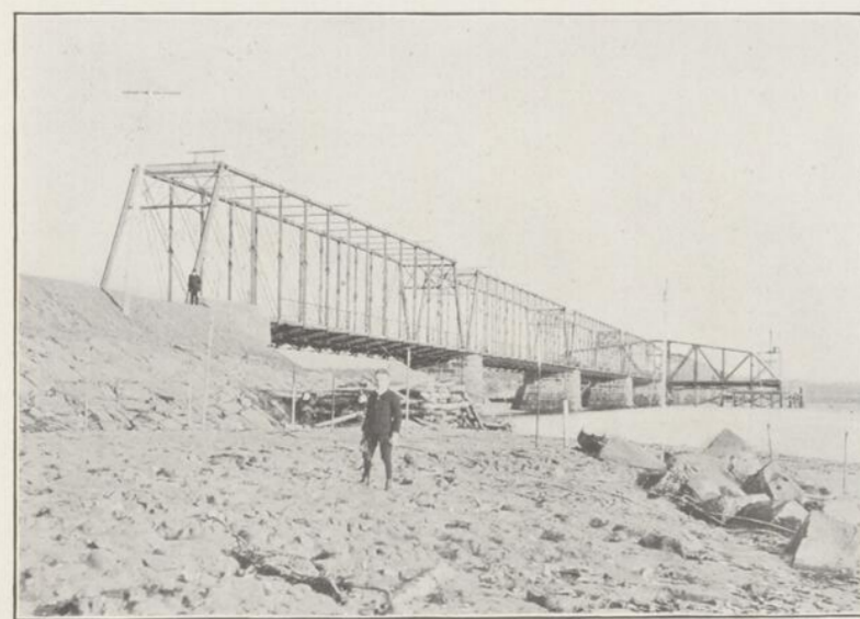
The newly completed bridge over the Hillsboro River, P.E.I. (First picture taken.)
