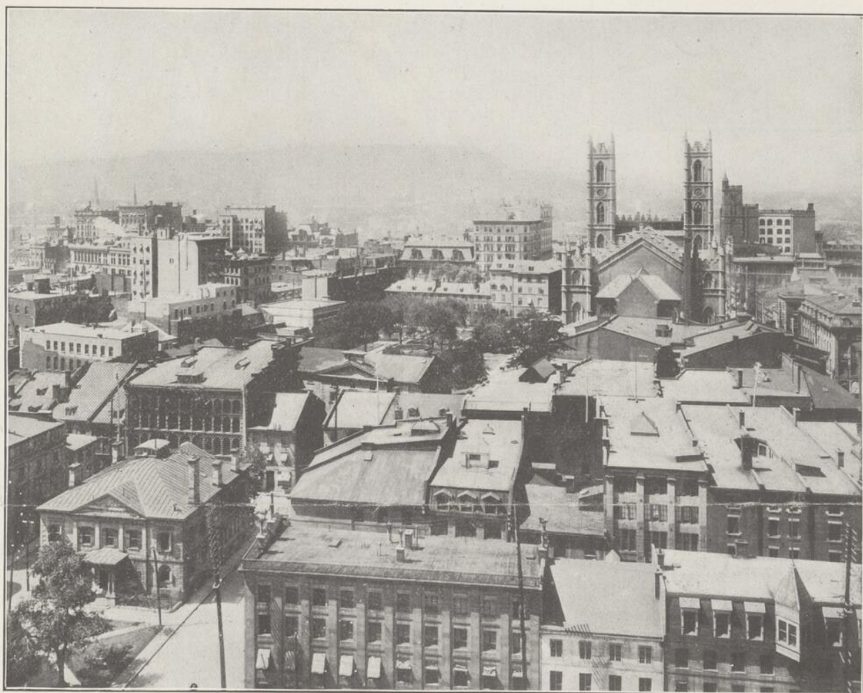
A VIEW OF NOTRE DAME CHURCH AND THE QUIANT OLD SEMINARY GARDENS Taken from the top of the Harbor Commissioners' Elevator. (Photographed for THE STANDARD.)
