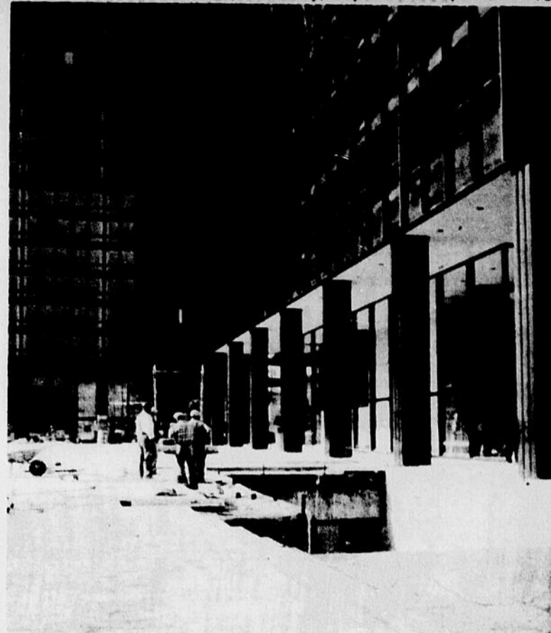
Westmount Plaza begins to shape up as one of the most attractive complexes in the area. Workers have cleaned up much of the rubbish that has been evident in the last few months.
