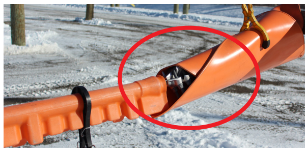
Incorrectly superposed conductor covers
