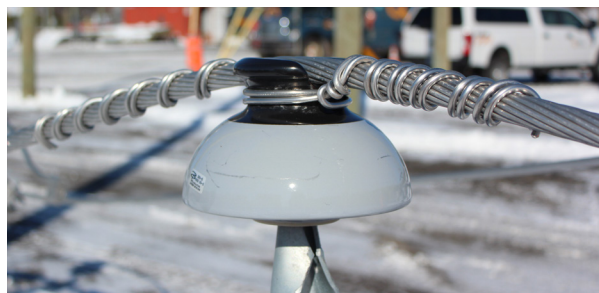
Tie wires in good condition
