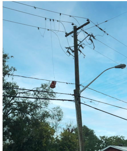
Grounding to de-energize part of a medium-voltage line
