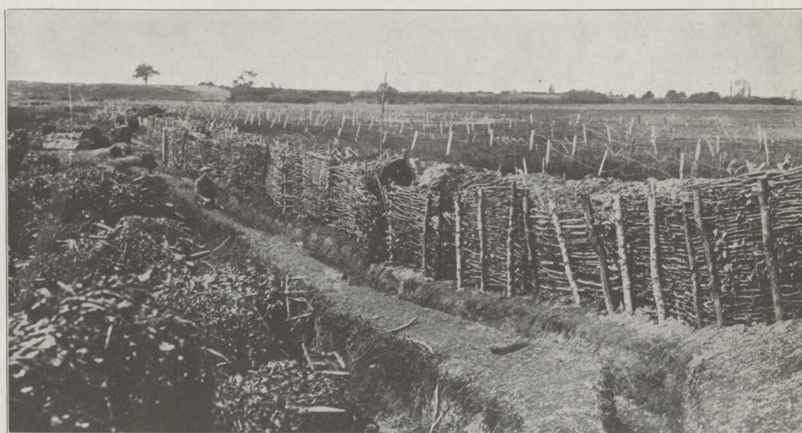
WHAT A MODERN BATTLEFIELD LOOKS LIKE. —A French first line trench near the Aisne showing the gabions and the barbed wire entanglements. —Photo Service of the French Armies.
