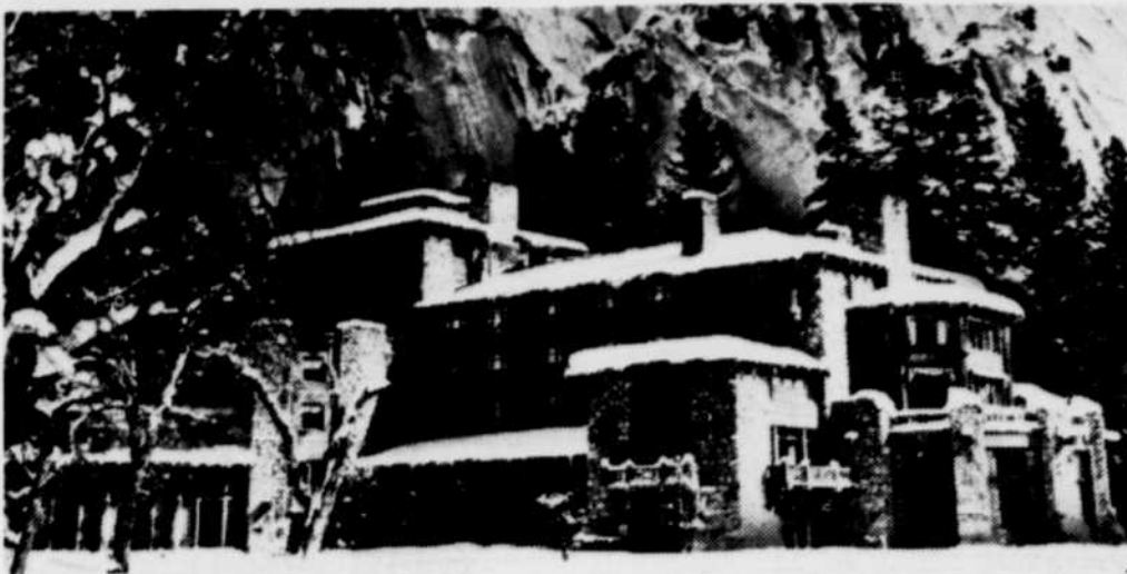
IN SPITE OF its paper-thin walls, cacophonous plumbing and walls of simulated timber, Yosemite's Ahwahnee Hotel demands, and gets, coats and ties for males using their dining room.
