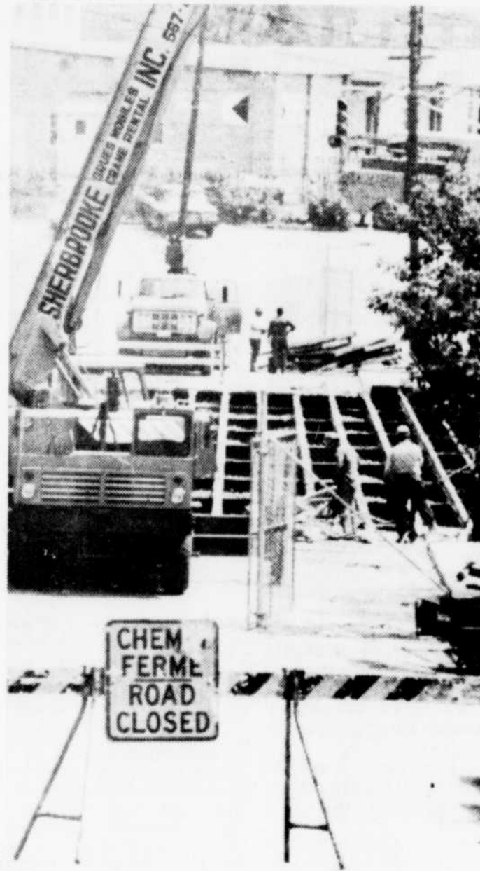
ROAD CLOSED — What's left of Wolfe Bridge is seen above as demolition work continues ahead of schedule. Perhaps the bridge will be open before July, 1977.
