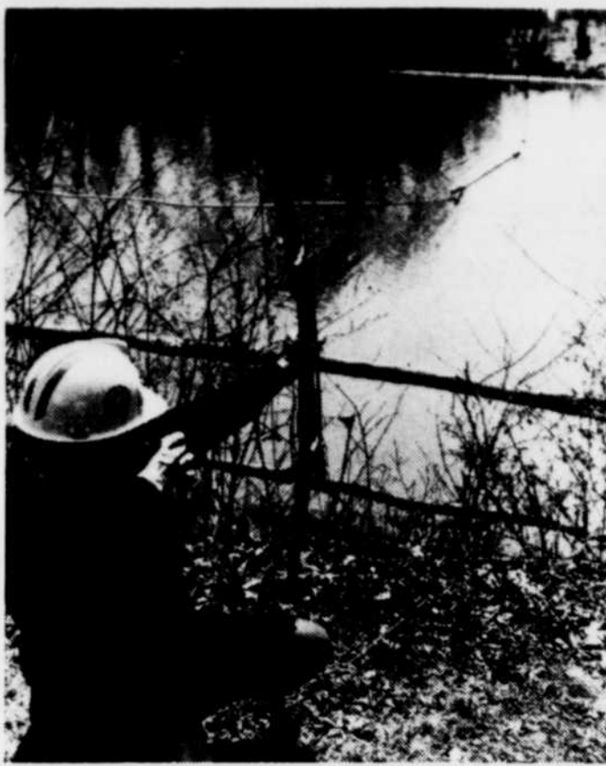
HE AIMS to restore phone service in a northwestern Ohio area. When floods snapped a riverbed cable and posed the problem of how to get a new line across the swollen Sandusky River near Tiffin, cable splicer Mel Jacobs came up with the answer in his 51-pound hunting bow. A nylon line attached to the arrow was the first step in stringing a new aerial cable across the deep river. Right, Ohio Bell crewmen Del Rice and Don Jackson anchor the cable to new poles.
