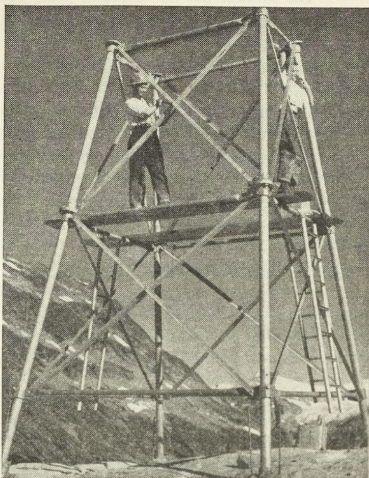
Tower for Alcan's test span under construction Towers are of aluminum.
