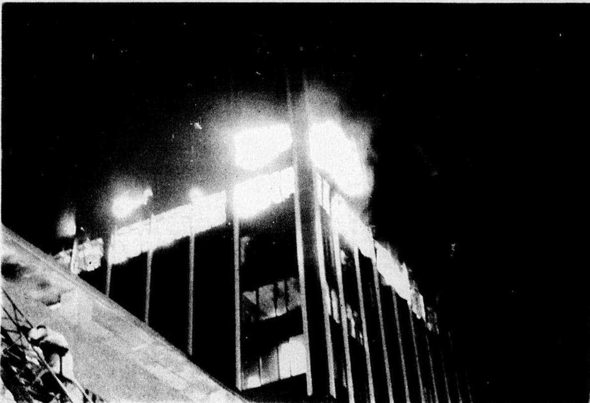
Oct 26, 1986: Multi-million-dollar fire sweeps through tower of Alexis Nihon Plaza .
