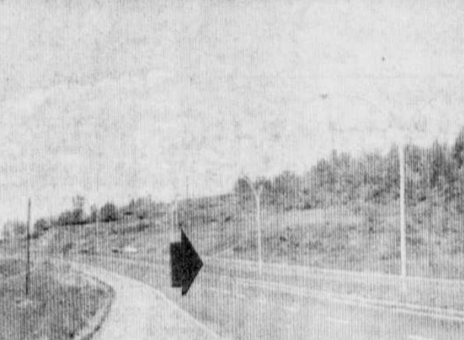
GOUIN PARK — Is the piece of land, to the right of the photo. The arrow shows where the access road from Adam Street led into the area. Now this roadway has been cut off by the new bypass on Route 22-32 leading to the new bridge crossing the St. Francis River. (Record photo by Wm. H. Lunan)
