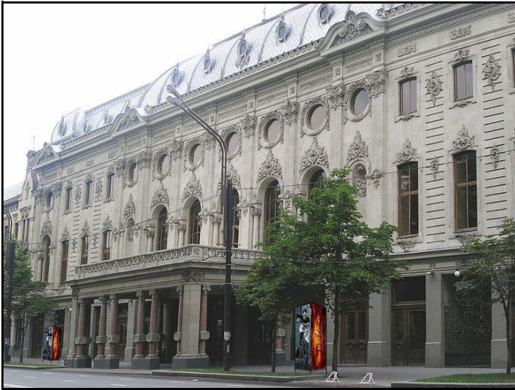
Figure 4.17: Theatre on Rustaveli Street.
