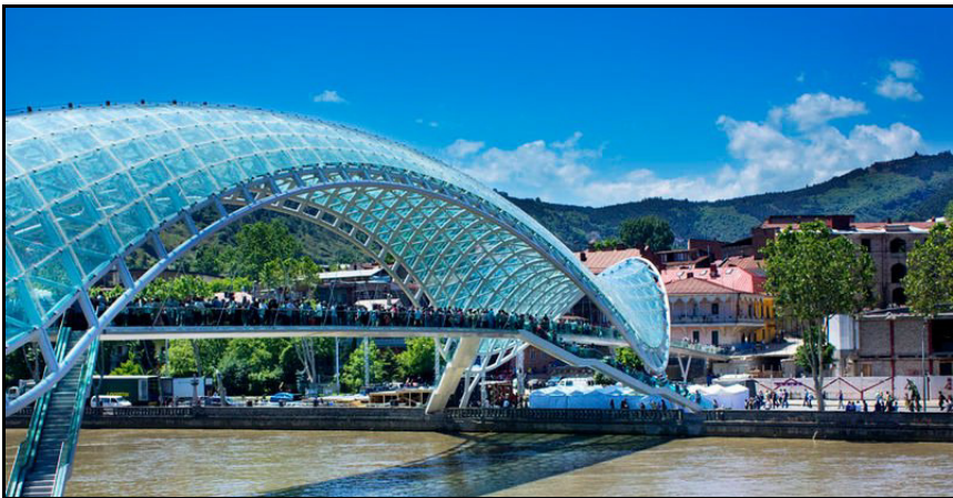
Figure 4.14: New bridge across Mtkvari River.
