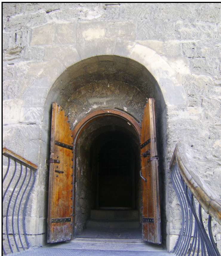
Figure 3.33: Entrance to the tower.
