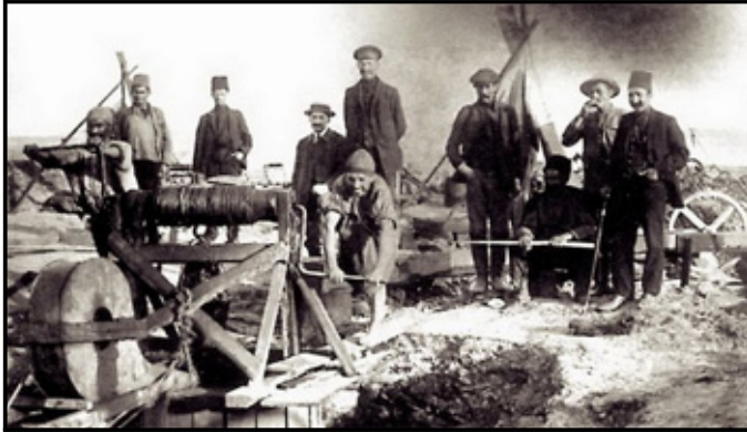
Figure 3.59: Workers in Baku using primitive drilling methods.
