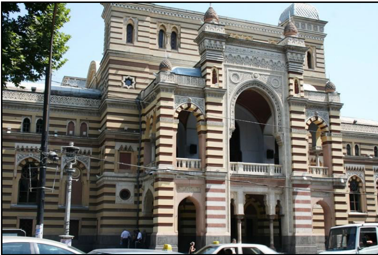
Figure 4.30: Opera House on Rustaveli Avenue.
