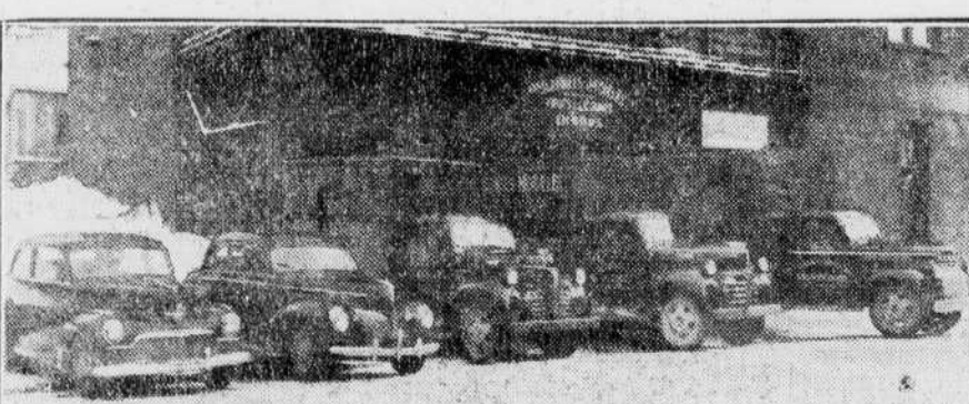
Our offices and warehouses at 6 Bowen North in Sherbrooke and fleet of trucks and salesmen's cars.
