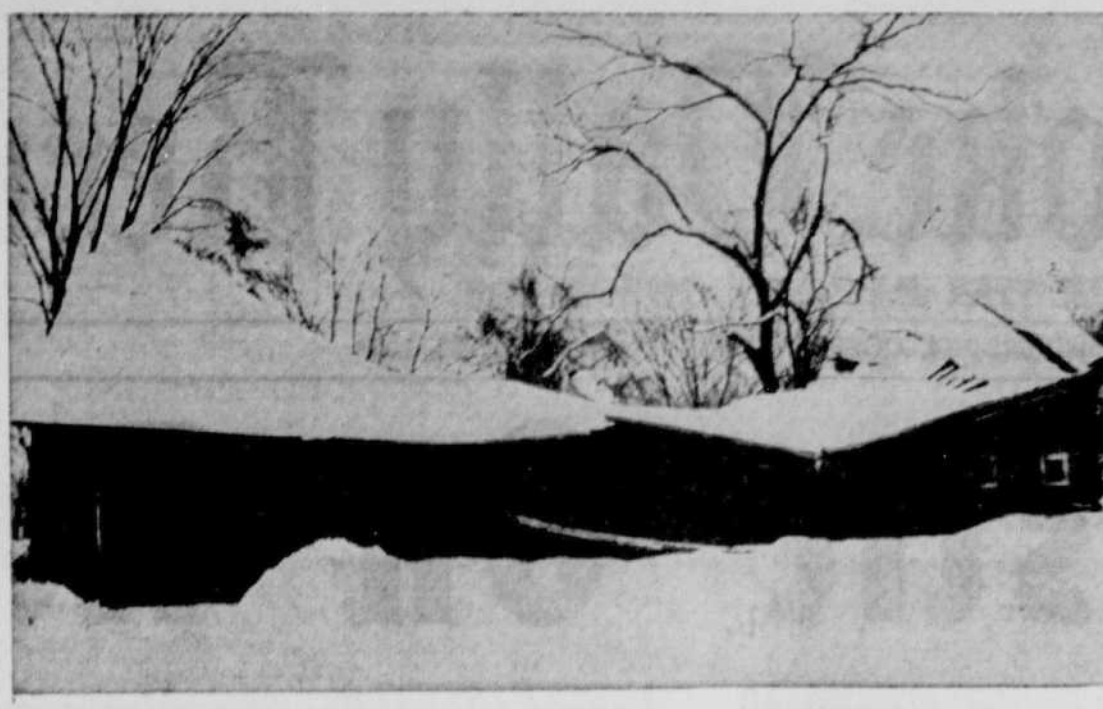
SNOW WRECKS BARN — This 40-year-old barn located at the Herbert Soutiere Farm near Tomfobia collapsed under the weight of snow Friday afternoon. The barn was built in 1919 for Peter O'Leary. (A. Pepin Photo)
