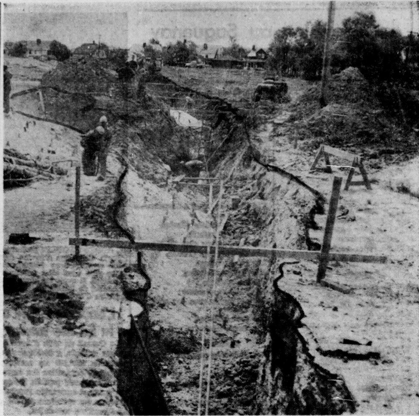
ROAD CONSTRUCTION crews prepare rock for St. The extension of three streets in this area will blasting on the extension of Ampere St. to Lavoisier create 48 lots for housing.
