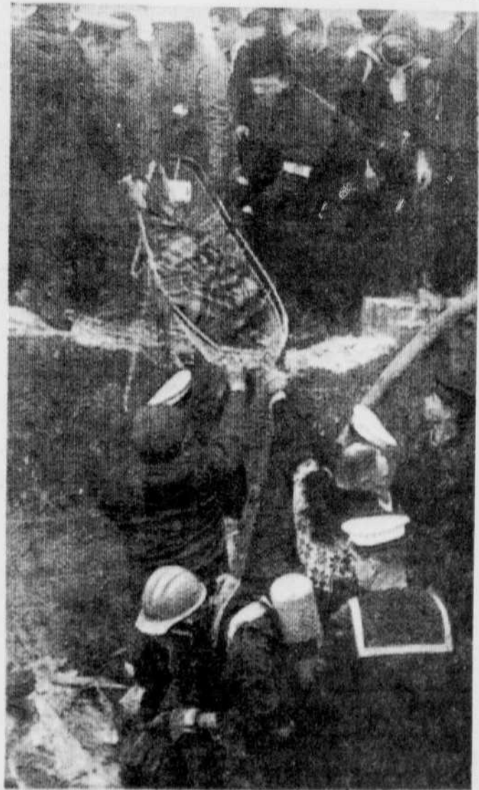
BODY REMOVED — A child's blanket covered body is seen here being removed from the wreckage of an apartment destroyed by an explosion in the Montreal suburb of LaSalle about 8:15 a.m. yesterday. The body was one of many found in the wreckage of the three-storey apartment. (CP Wirephoto)
