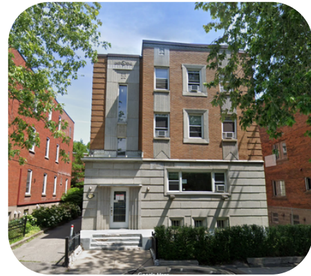
Google Maps, 1475 Morgan, construction 1951
