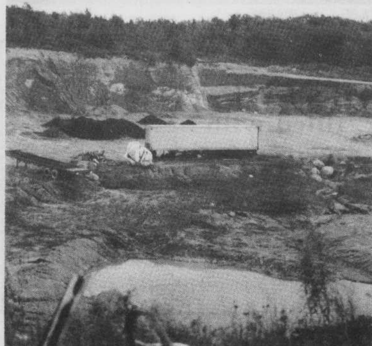
Experts disagree on effectiveness of plastic membranes at landfills
