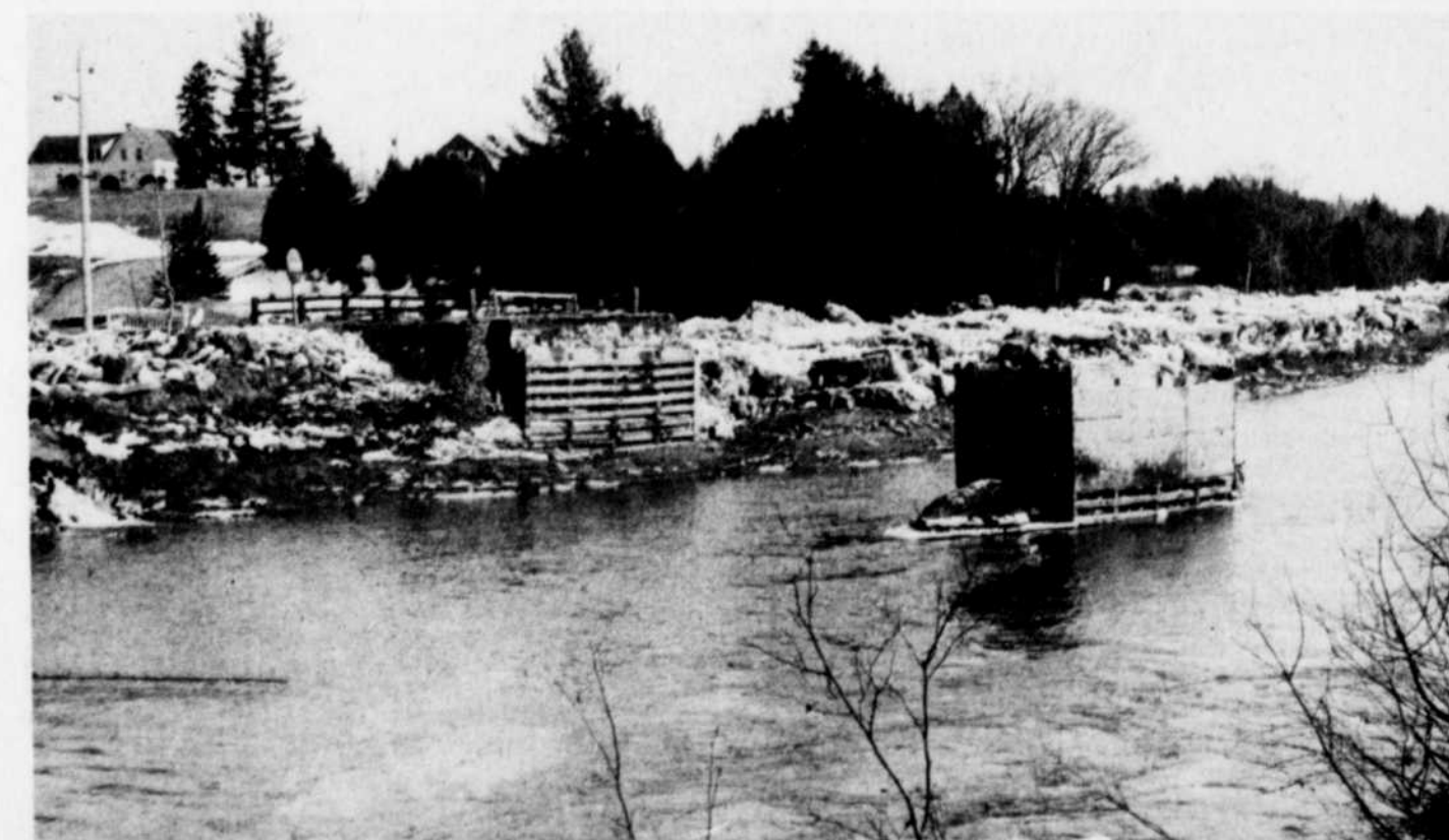
BRIDGE GONE — The Bower Bridge across the Salmon River at Milby is no more but the flood waters have subsided and the residents across the river are safe. However, the opening of the
