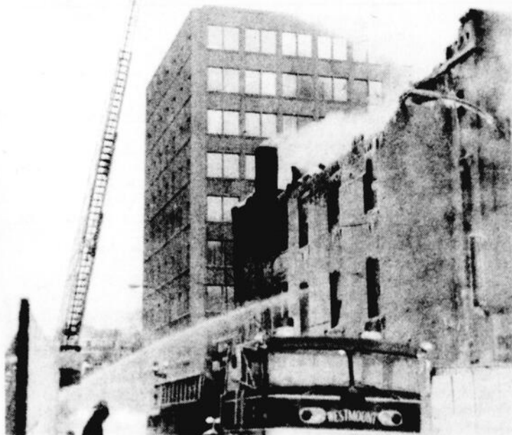
The scene up Victoria avenue as the fire died down after 7:30 am shows the extent of damage to the outside of the building.
