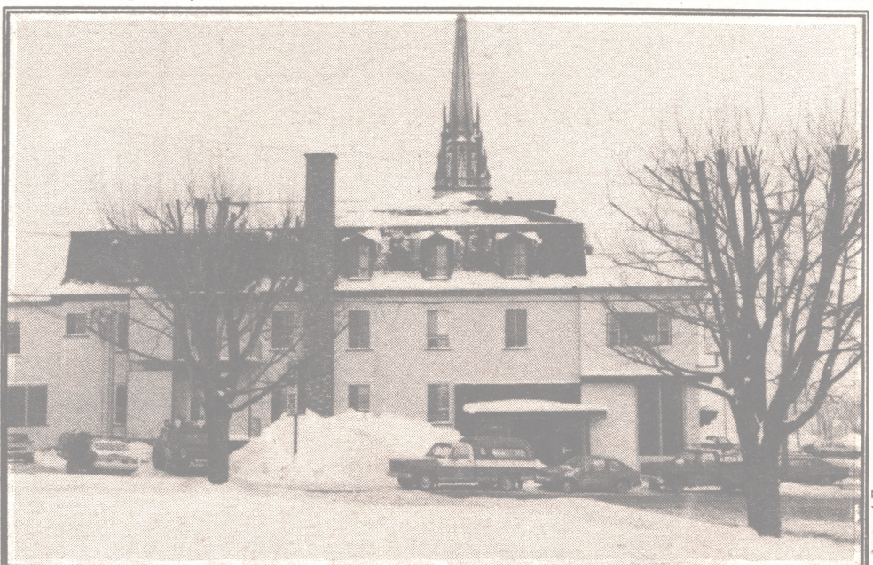
The Angus House as it stands today. Note the Catholic Church in the background in the 1896 photo also.
