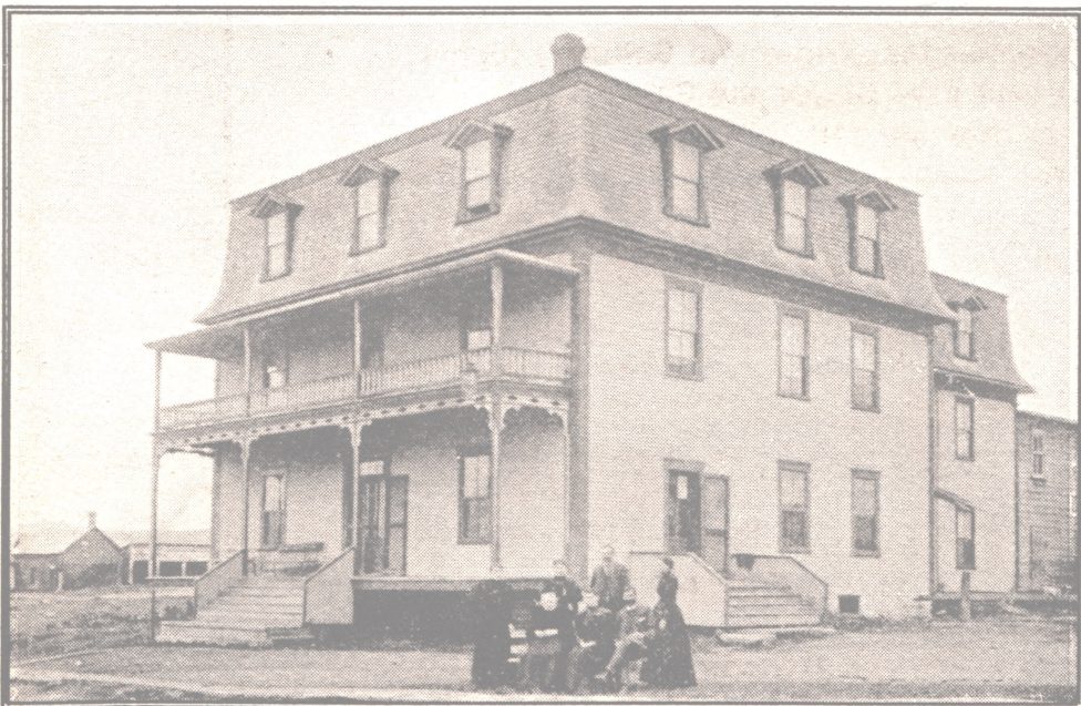
Angus House was an elegant hotel in its day. Built in 1891 by James Bryant, owner of a local boarding house, it was sold to L.R. Willard of Sawyerville.
