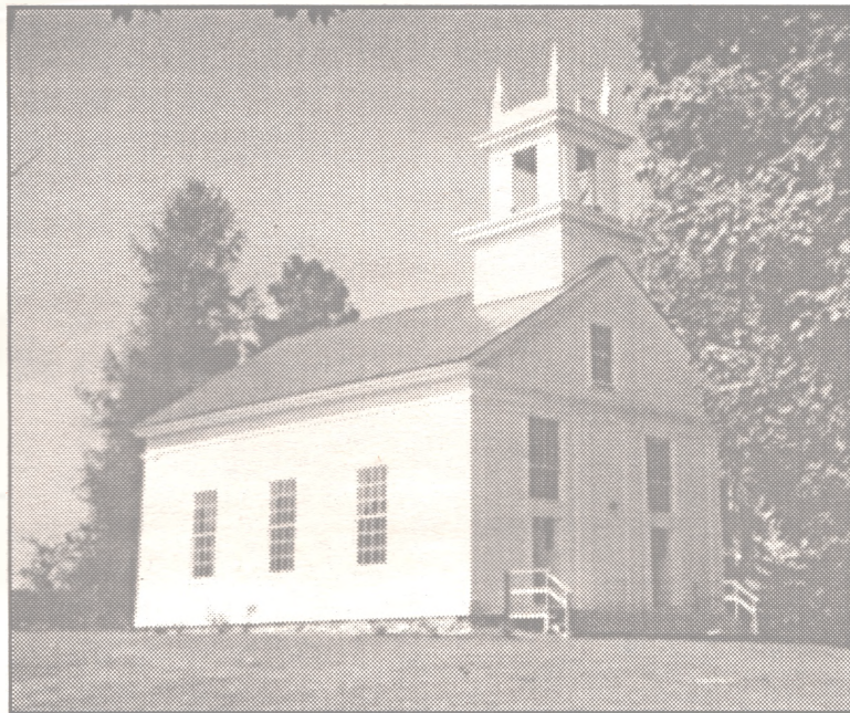
The newly-renovated Huntingville Universalist Church.
