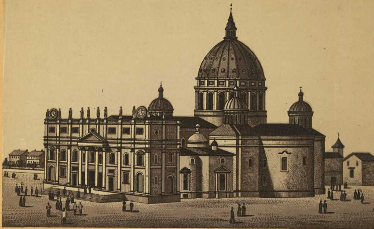
EXTERIOR OF ST. JAMES CATHEDRAL.
