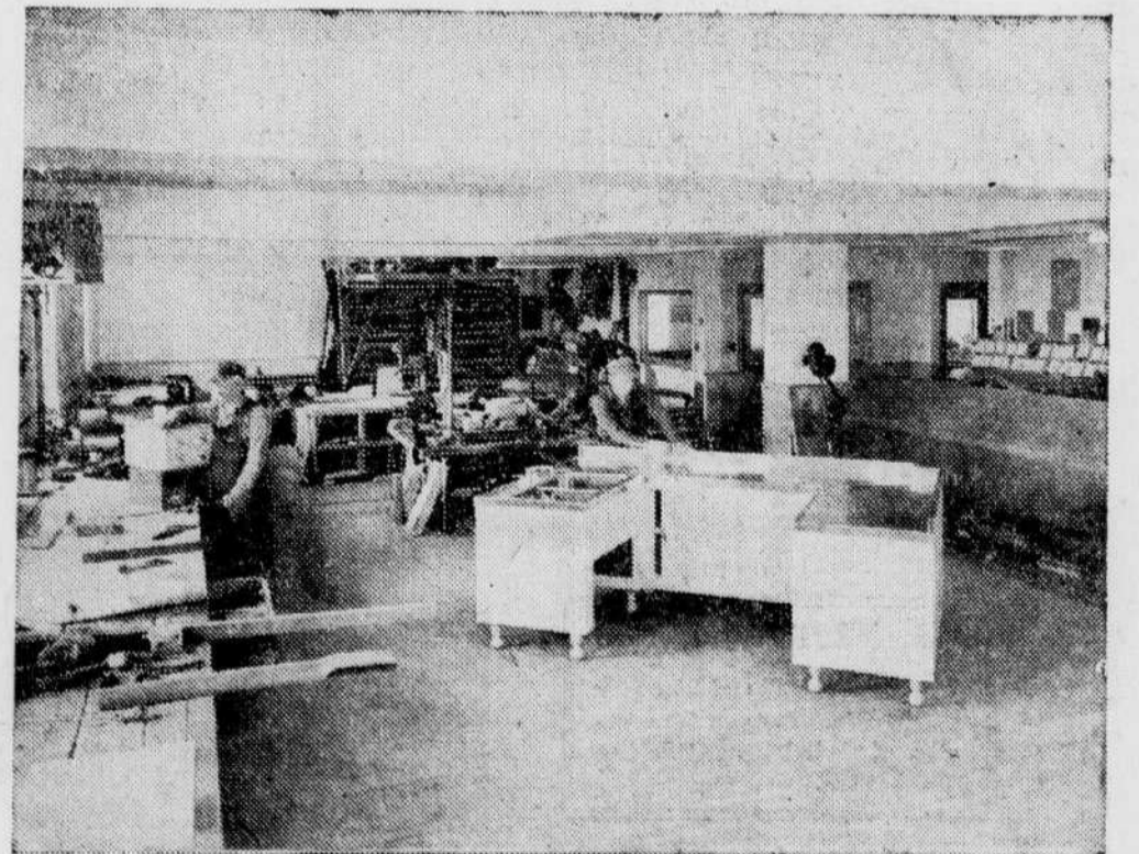
METAL SHEETING SHOP
