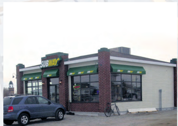
Construction Subway - Havre St-Pierre.
