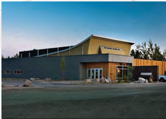
Construction centre commercial Pessamit.
