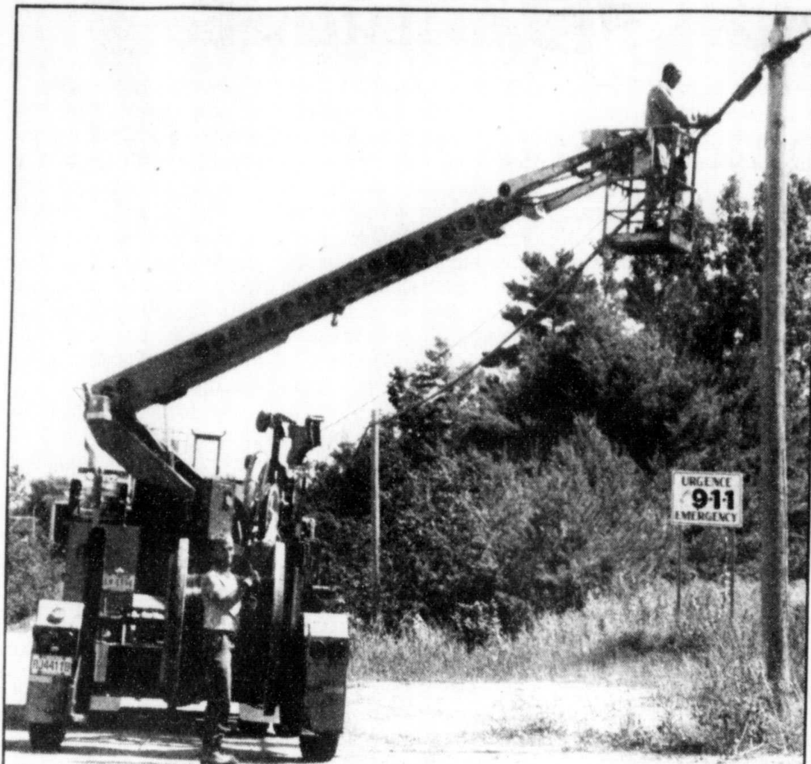
STRINGING CABLE: Regional Cable is replacing its lines in Pontiac to improve reception and offer cable Internet access. Workers are seen here stringing cable near Shawville recently.
