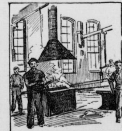
FORGING AN ENGINE FRAME.
