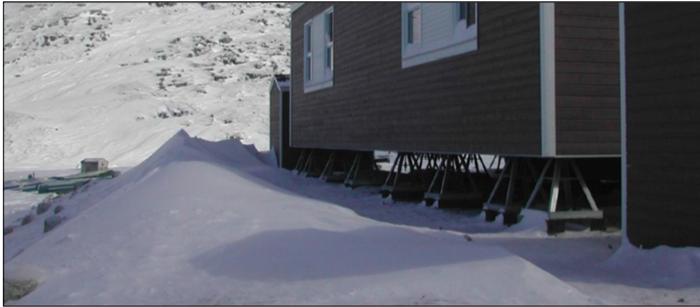
FIGURE 3.1: HOUSE CLEARANCE ABOVE GRADE / SOURCE: SHQ
