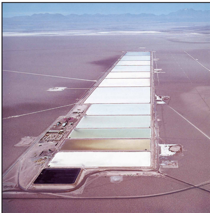
Figure 8.8.8 - Brines containing lithium is pumped from underground to the ponds for concentration by evaporation in Atacama Desert
