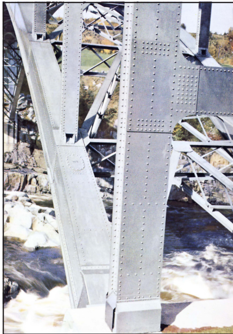
Figure 8.10.40 - All-aluminum highway bridge near Arvida, Canada
