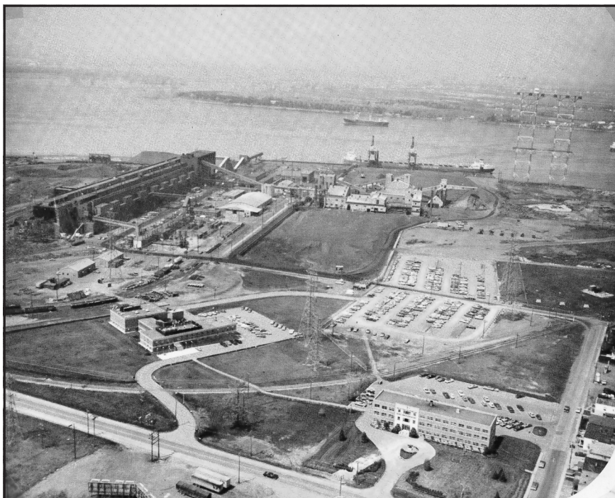
Figure 7.10.14 - QIT Fer et Titane plant at Sorel, Quebec. Electric furnaces are in the building to the left; facing the building are piles of anthracite and ilmenite and mineral beneficiation plant. The river at the top of the photograph is Saint Lawrence River
