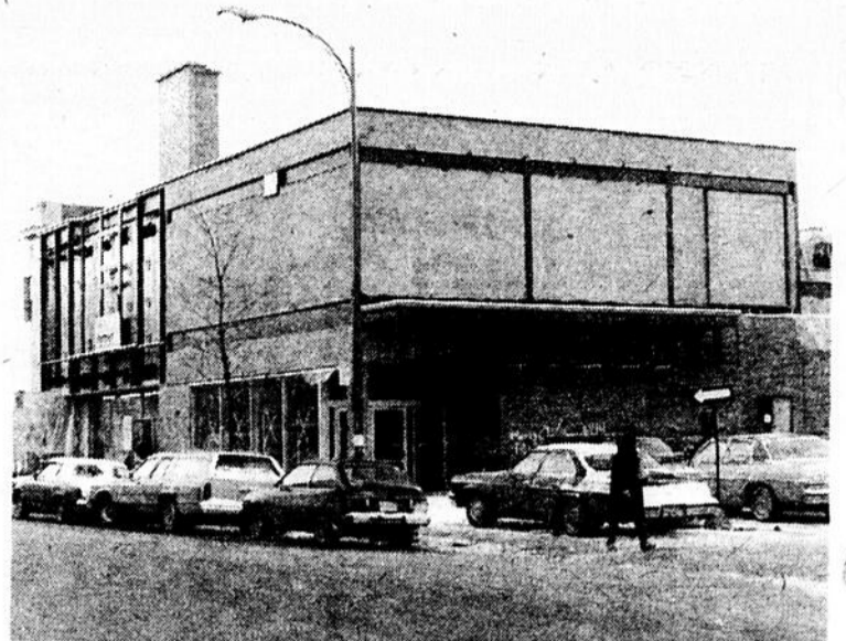
PROGRESS: The new extension to Steinberg's Victoria avenue-Sherbrooke street outlet has been closed in and the parking lot completely reopened, according to store officials. The wing will be completed by early February, and crews then will begin renovating the existing part of the store, working on nights and weekends to try to disrupt regular users as little as possible. The entire renovation is expected to be completed in April.
