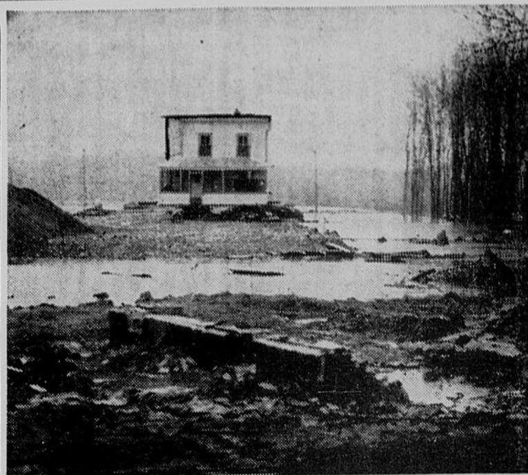
This house has been on the move since last fall to make way for the approach to the bridge across the Chateauguay river connecting the new road from Woodlands to the Mercier Bridge. This is the south side of the river. Work for the bridge is actually underway on the other side of the river. (Photo by Pat Wilkins)
