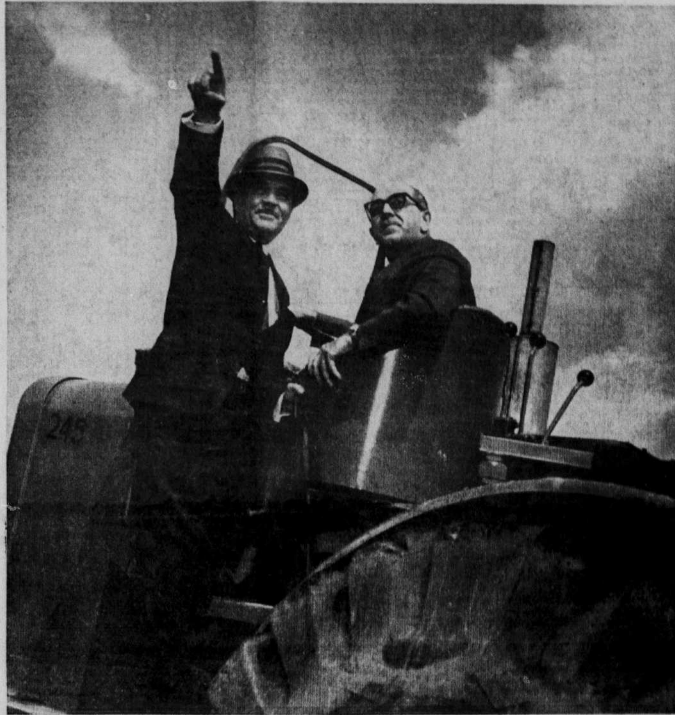
AUTOROUTE CEREMONY — Guy Poliquin, left, president of the Quebec Autoroutes Office, and Carrier Fortin, minister without portfolio and Sherbrooke MPP, are mounted on an earth-moving machine for ceremonies marking the start of construction on the Eastern Townships Autoroute yesterday at Omerville.
