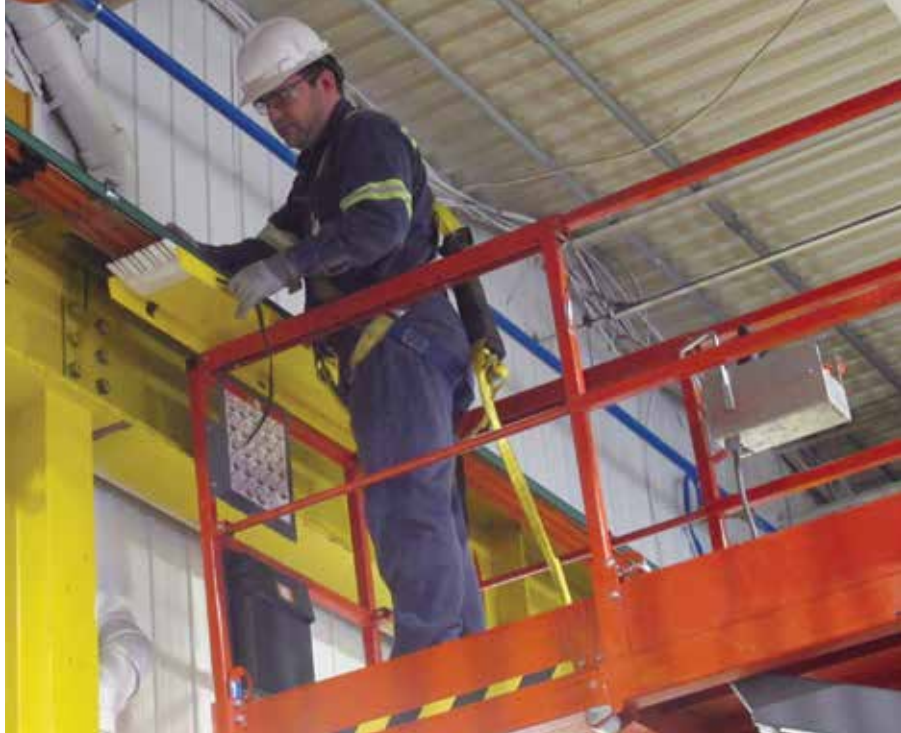
Source : Fives Services Inc.
