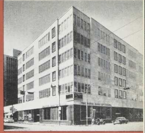
Immeuble Royalite Oil Architectes : Rule, Wynn & Rule Entrepreneur : Poole Construction Co.
