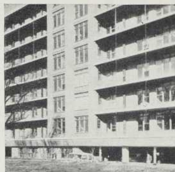
Park Tower Apartments, Winnipeg, Manitoba. Entrepreneurs: F. R. Lount Construction Co.
