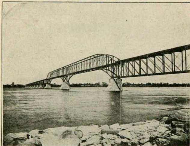
C.P.R. BRIDGE, LACHINE
