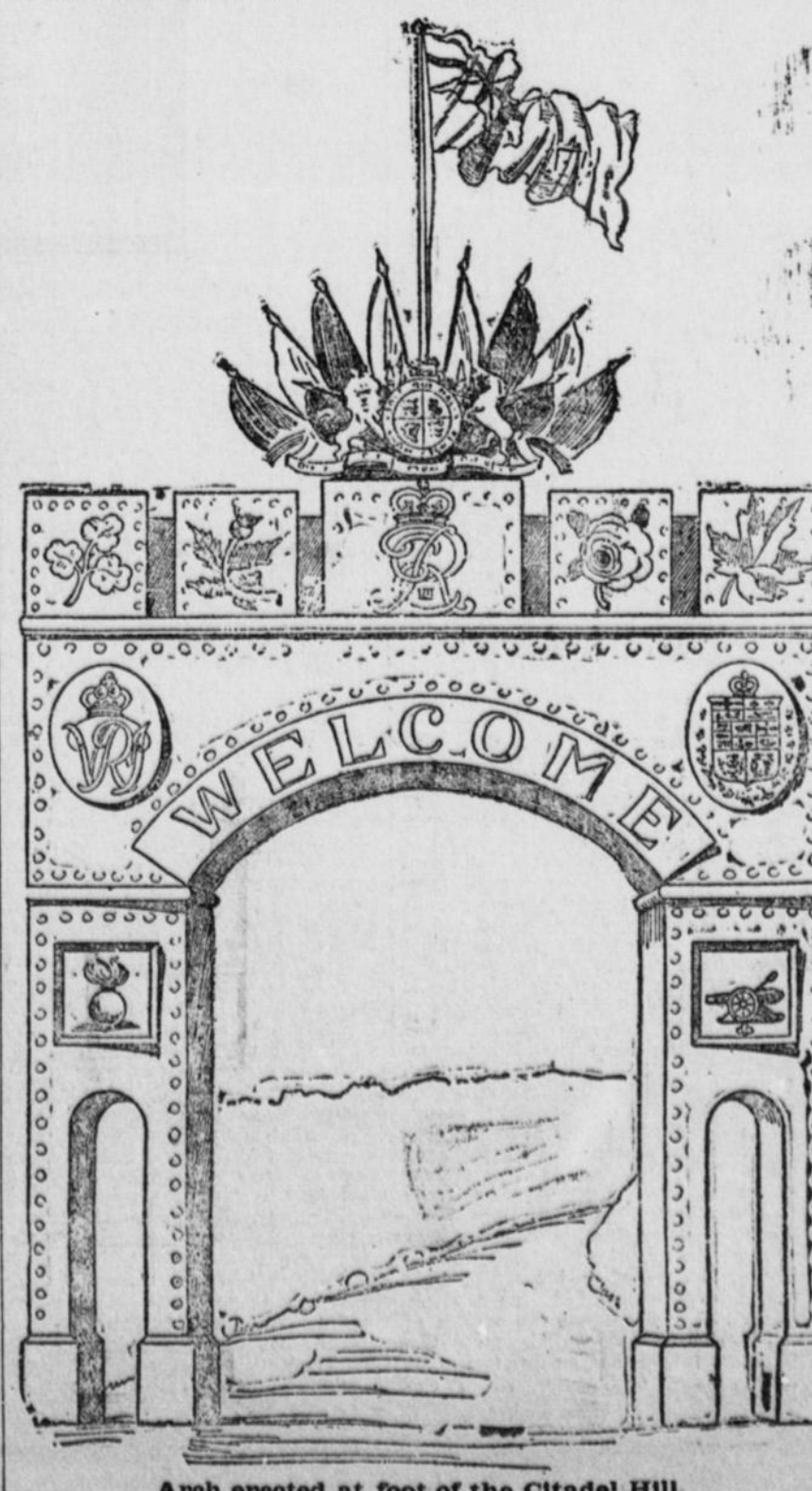
Arch erected at foot of the Citadel Hill.
