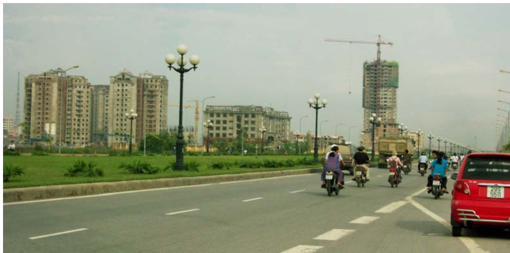
Figure 7.3 High-rise buildings under construction on the western edge of Hanoi Source: D. Labbé, 2005
