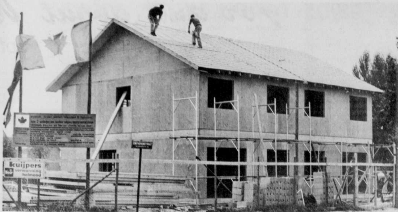
BUILDING THE CANADIAN WAY — Workmen build a two-storey house near Eindhoven in The Netherlands using Canadian timber-frame technique and British Columbia hemlock and fir plywood and Western Red cedar. The Canadian government has been trying to interest Western
