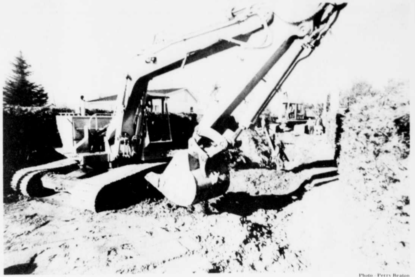
Installation of the sewage-water system at Plage Southiere got underway Tuesday.
