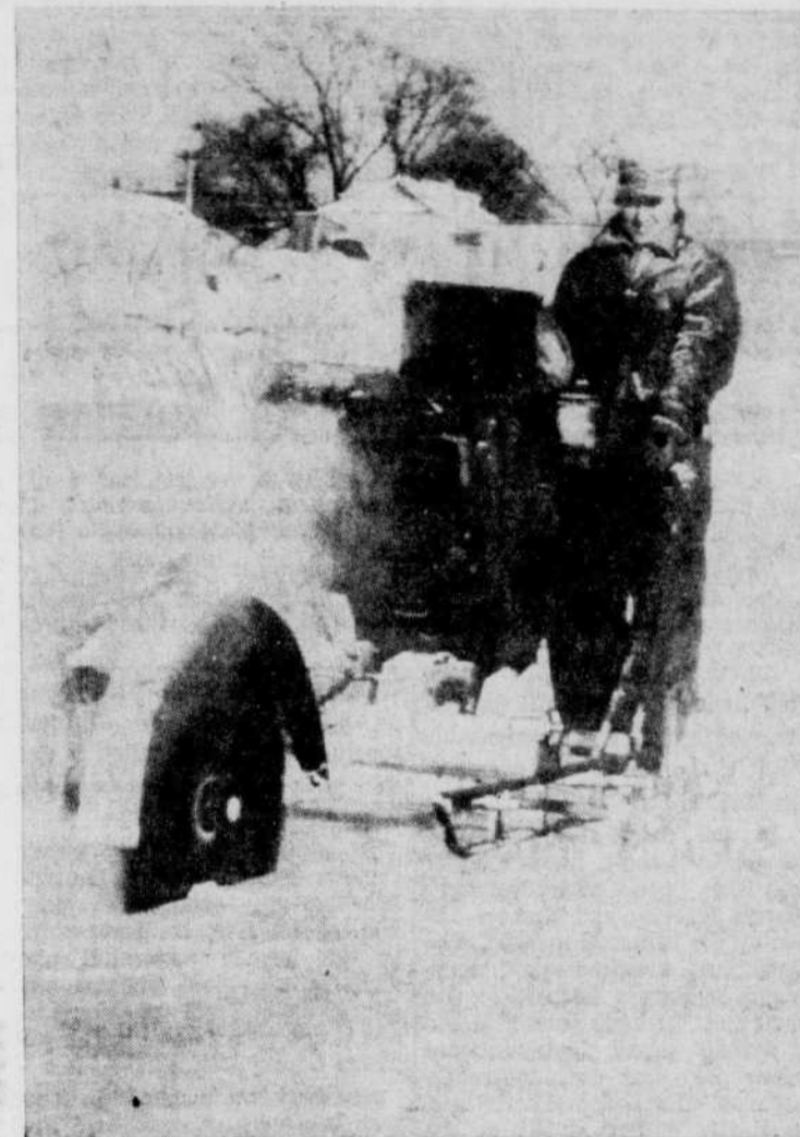
Cutting ice from the Magog River is done by a gas-operated saw. Mac Ross, son of one of the owners of the Sherbrooke Ice Company, is shown cutting the 17-inch thick ice into blocks 22 by 36 inches. A 15-acre lot was cleared by the company three weeks ago and operations should be completed this week-end, when all three ice-houses are filled.
