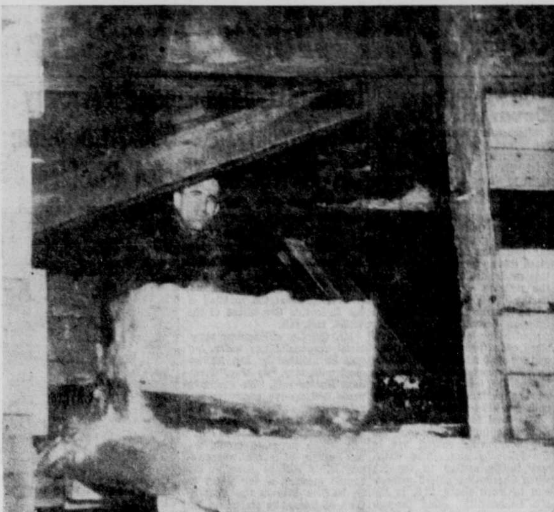
Directing ice down the ramp into the ice house is Roland Alexandrini, who keeps the cakes from falling off the end of the chain as it turns into the building. When the three Esplanade Street ice houses are filled, 500,000 tons of ice will be stored away for the months ahead.
