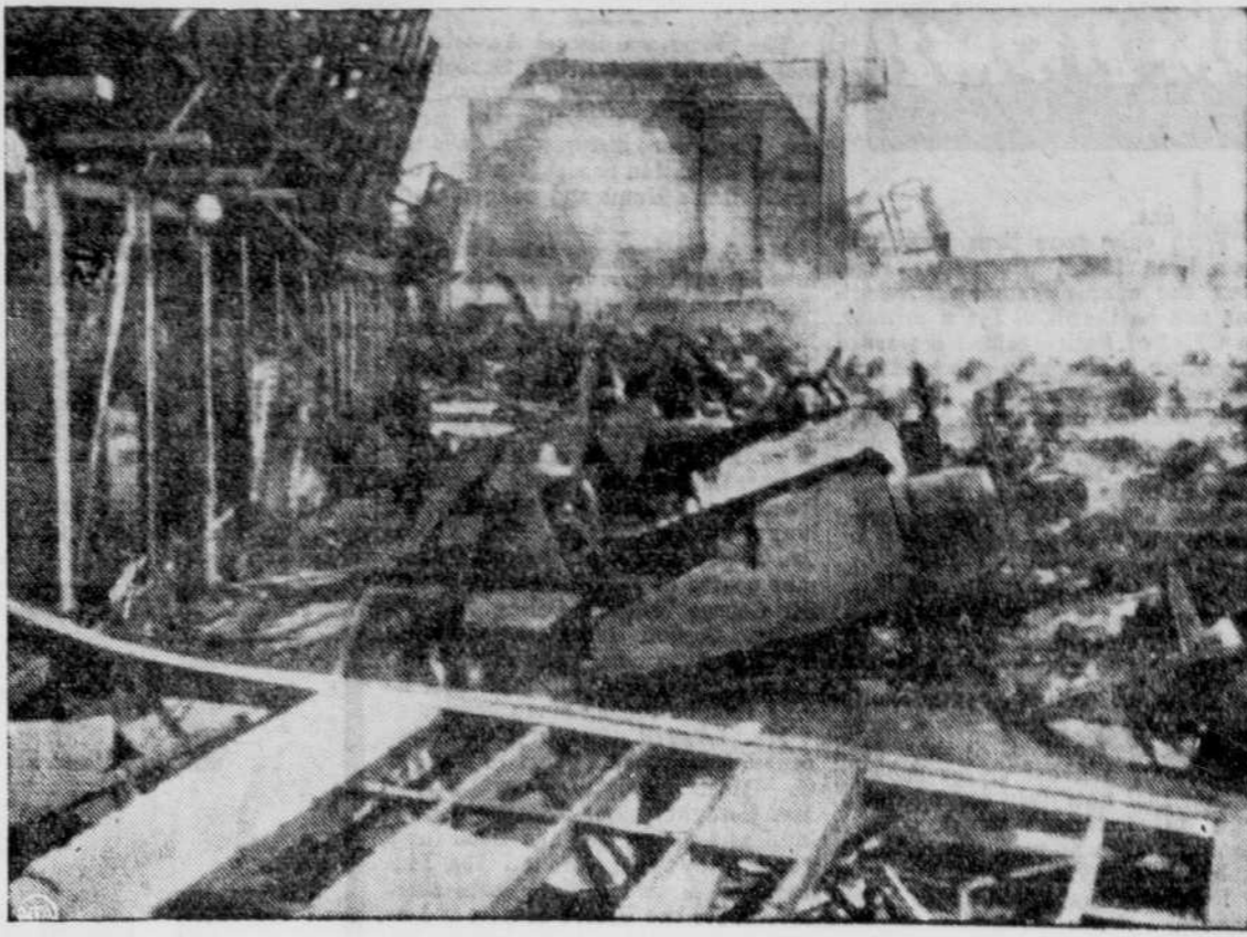
Smoke drifts from the smouldering wreckage of 366 U. S. Navy planes which were destroyed at the Richmond Naval Air Station when a hurricane struck Miami, Fla. Storm winds collapsed the roof of three huge hangars setting fire to the planes and 25 patrol blimps. Loss at the base alone was estimated between $30,000,000 and $40,000,000.
