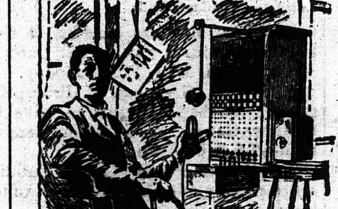
INTERIOR OF TELEPHONE OFFICE.
