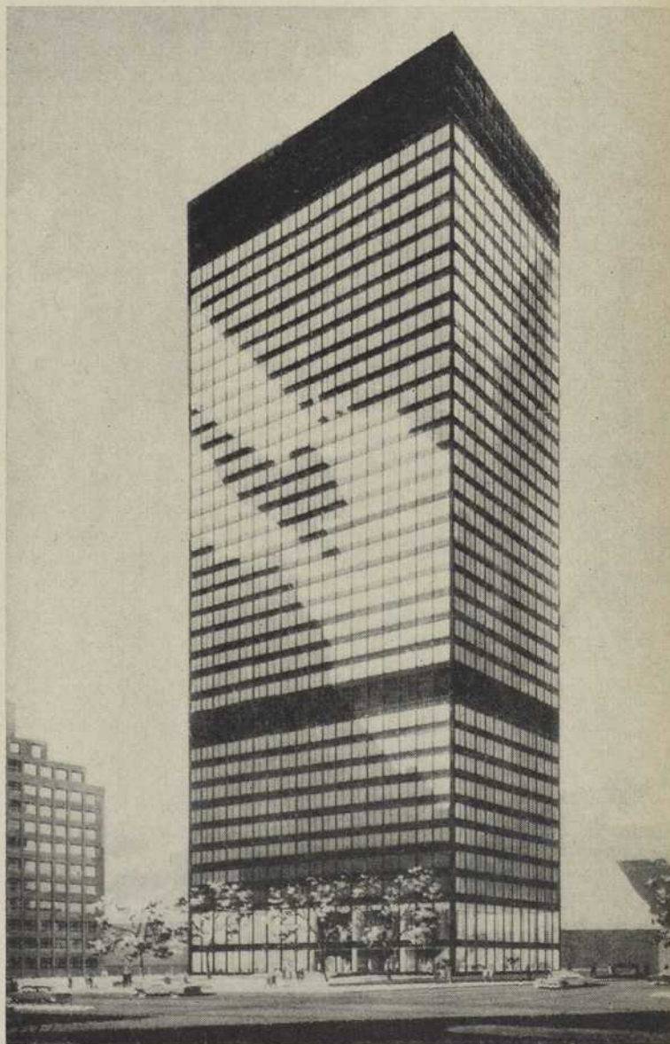
VIEW OF THE NEW C-I-L HOUSE AND OF THE PLAZA FROM DORCHESTER BOULEVARD AND UNIVERSITY ST.
