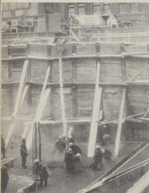
POURING THE FIRST CONCRETE IN THE EXCAVATION OF THE NEW C-I-L HOUSE NOW UNDER CONSTRUCTION.
