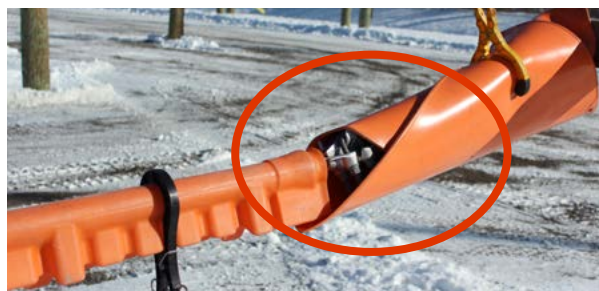
Incorrectly superposed conductor covers
