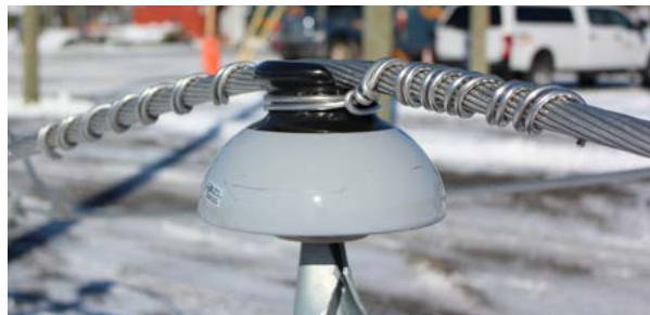
Tie wires in good condition
