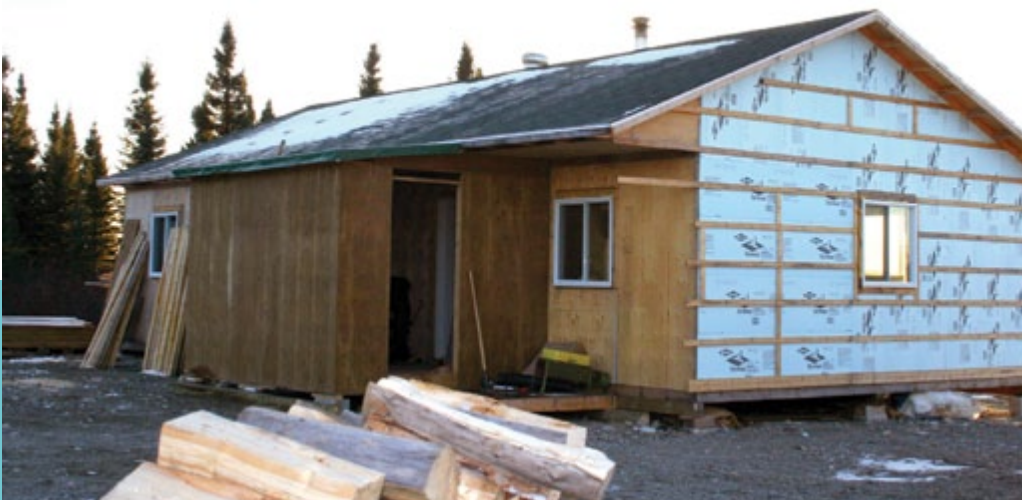
Camp under construction on Lac Mitsumis
