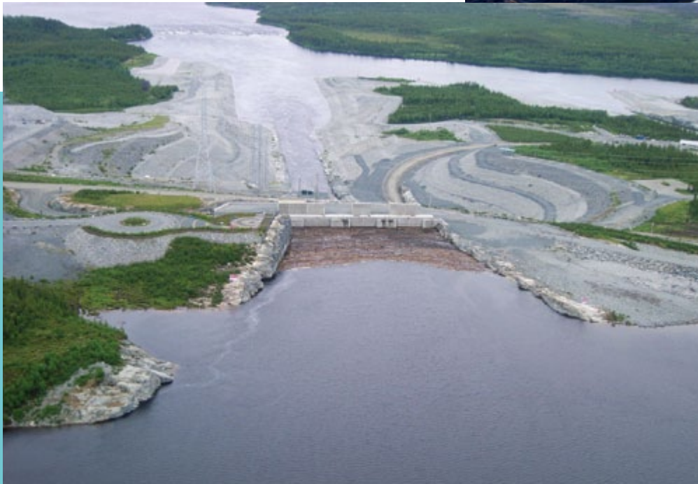
Wood debris at the Eastmain-1 powerhouse intake
