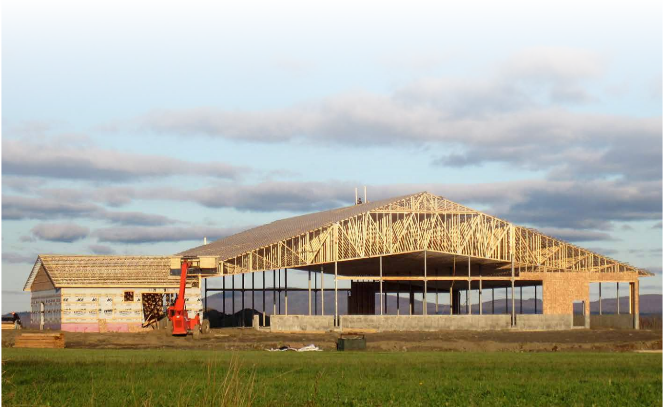
Wide-span wood prefabricated roof trusses, farm building. Photo: Structures RBR
