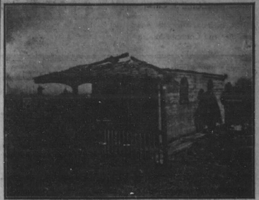
THE CABIN AS IT WAS A WEEK OR TWO AGO—ONLY THE FOUR WALLS NOW REMAIN
